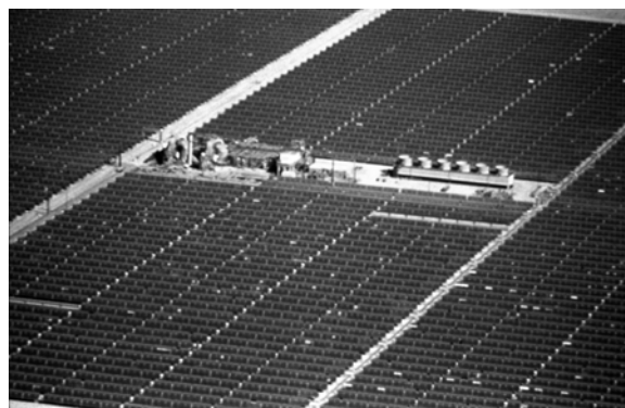
Figure 10-15 Parabolic-trough based solar thermal power plant in California (parabolic trough collectors [left]; power plant [right]) Source: Goswami
