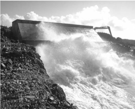
Figure 14-2 Shoreline OWC – the LIMPET
