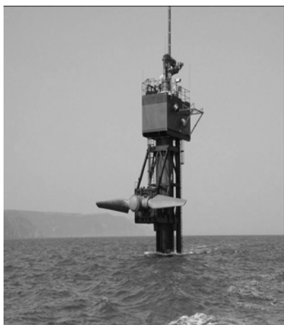
Figure 13-7 Seaflow with the nacelle raised Source: Marine Current Turbines
