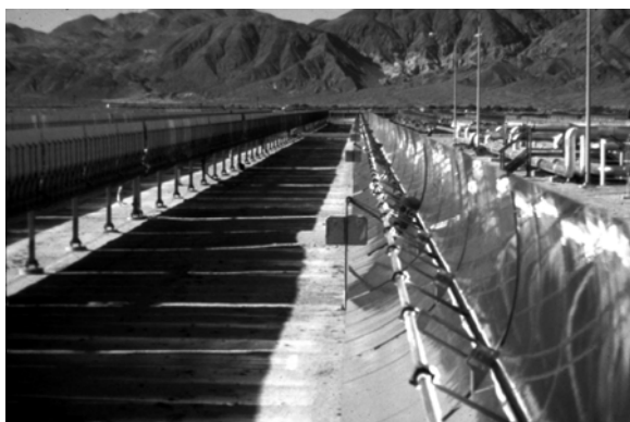
Figure 10-15 Parabolic-trough based solar thermal power plant in California (parabolic trough collectors [left]; power plant [right]) Source: Goswami
