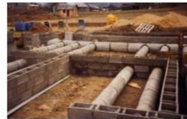
Soil-preheated air-heat pump
