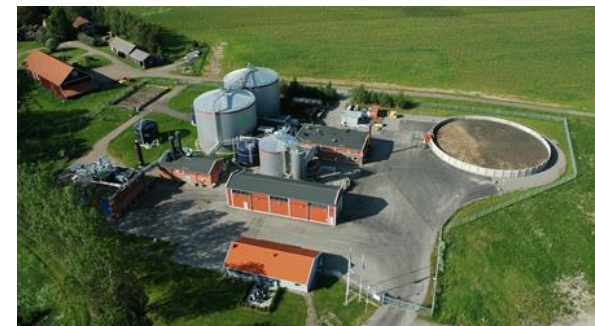
Biogas plant in Sweden, Linköping [Svensk Biogas, 2008]
