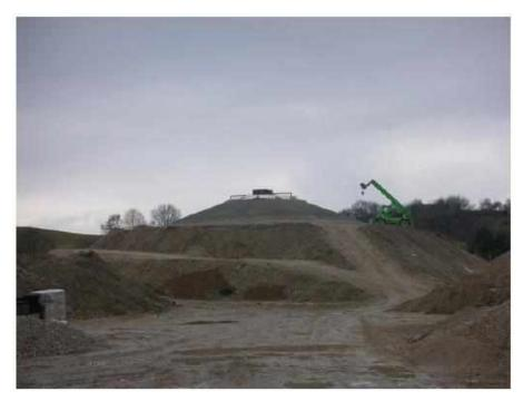
Figure: Sand layer at above ground TTES system
