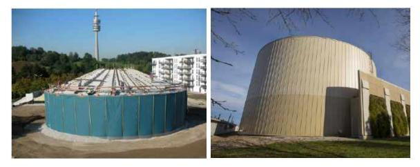
Figure 3-7: partially dug-in water storage tank (Solites) Figure 3-8: Water storage tank at Nebraska University
