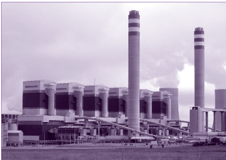
Figure 23 • Majuba power station
