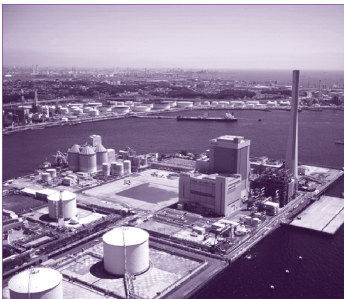
Figure 14 • Isogo New Unit 1 general view
