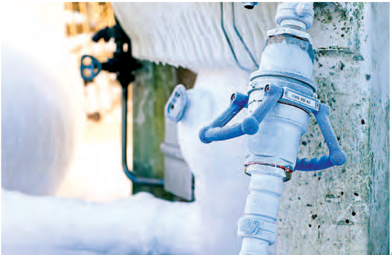
Figure 50: Example of a quick-connect coupling
