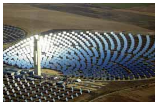
Source: ESTELA (central receiver technology)
