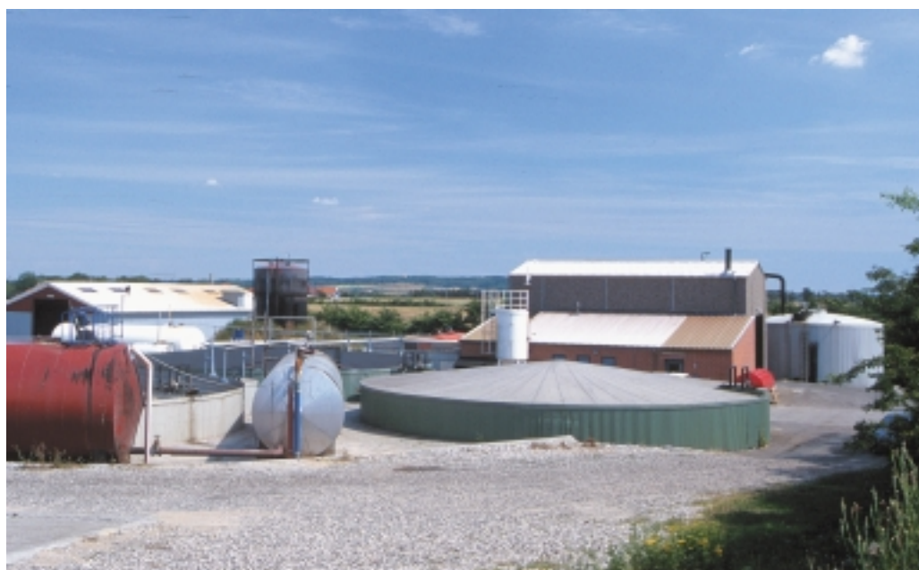
The Vester Hjermitslev plant is the oldest centralised biogas plant in Denmark, constructed in 1984. It is still in operation though biogas technology has developed considerably since then.
