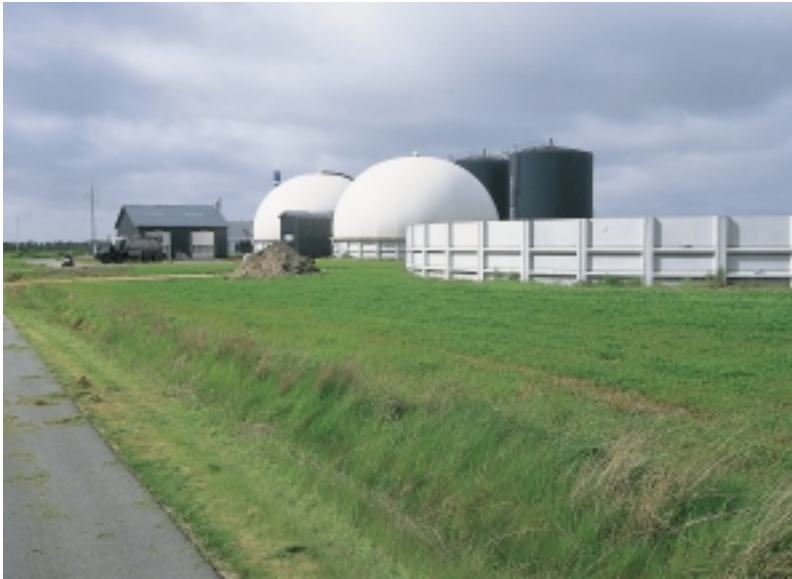
The Blaabjerg Plant was constructed in 1996, equipped with two low-pressure biogas storage facilities.
